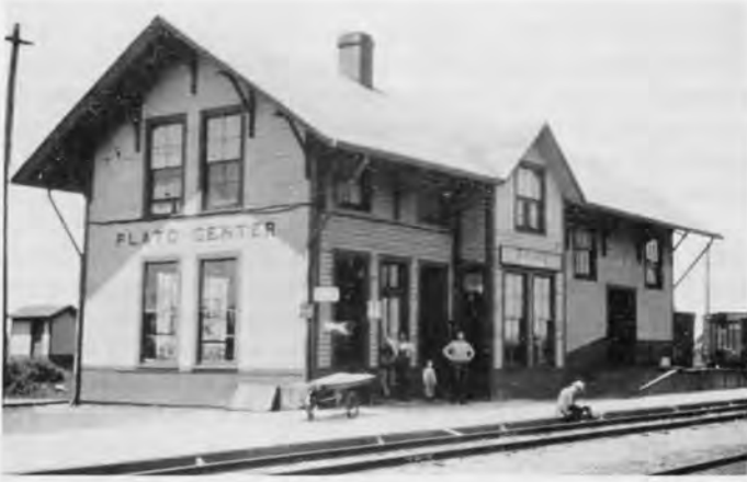
Plato Center Station.
