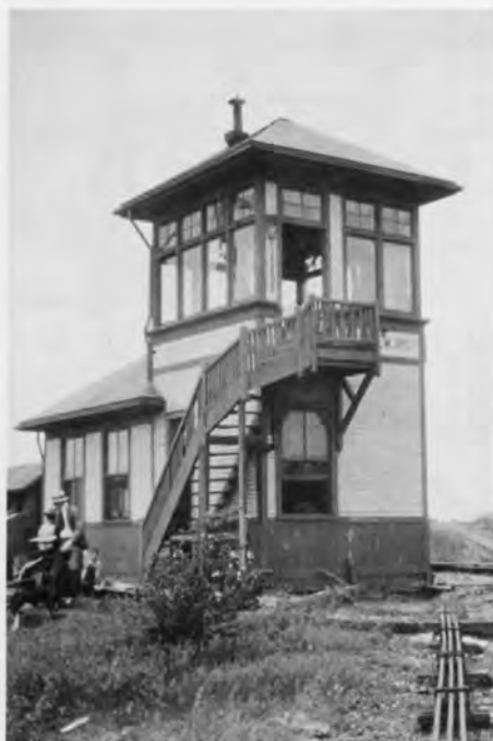
C&NW crossing tower.
