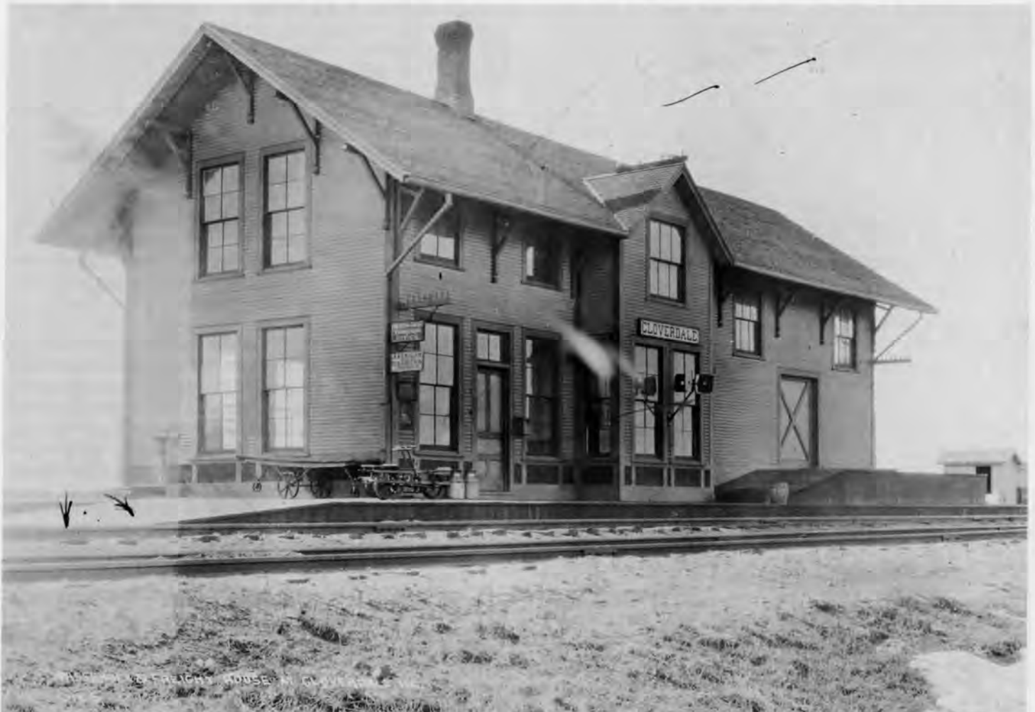
The Cloverdale (now Carol Stream) freight and Passenger house apparently soon after construction, (note the temporary train order signal. 2-25-1895. Valuation photos - ICHS Collection
