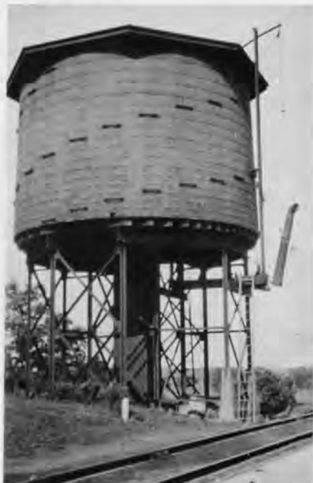
Water tank - Coleman.
