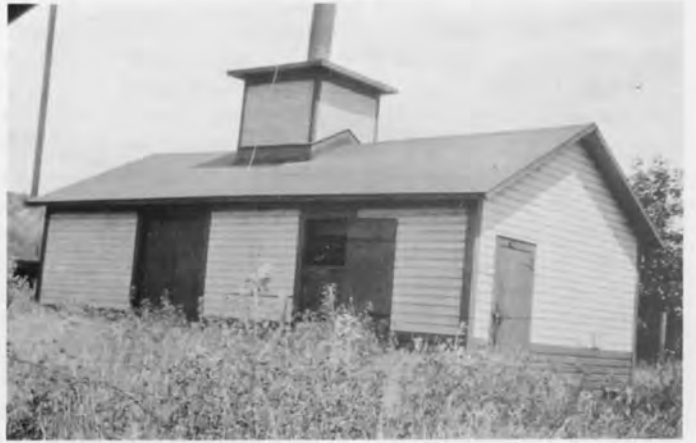
Hart pump house.
