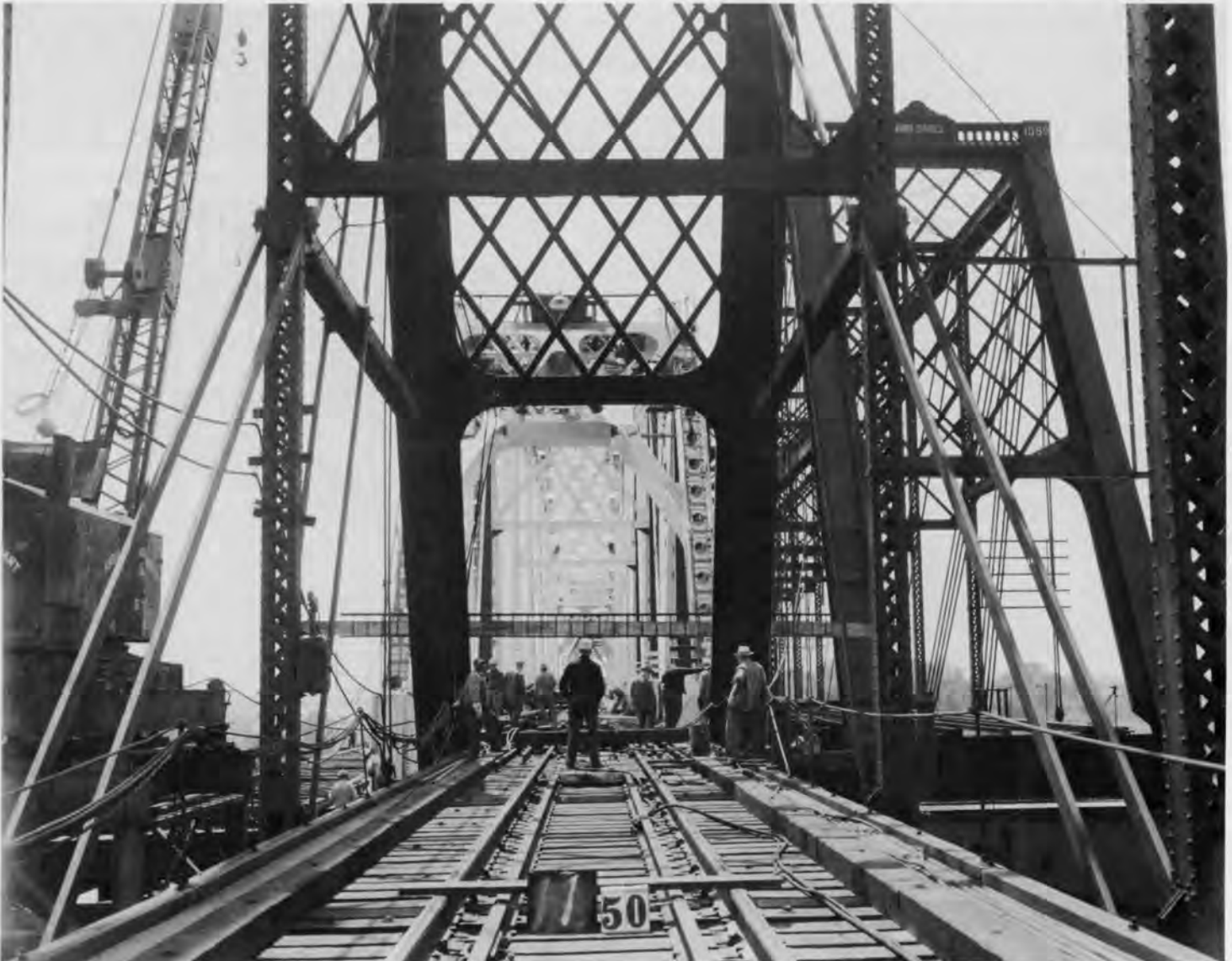
Almost there - the new span is moved into alignment.
