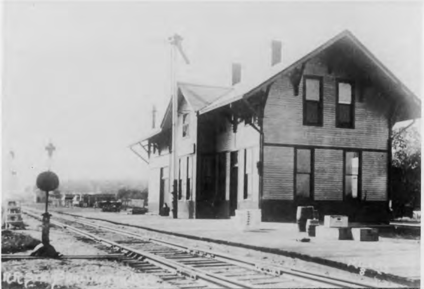
Illinois Central Station at Burlington, Illinois.
