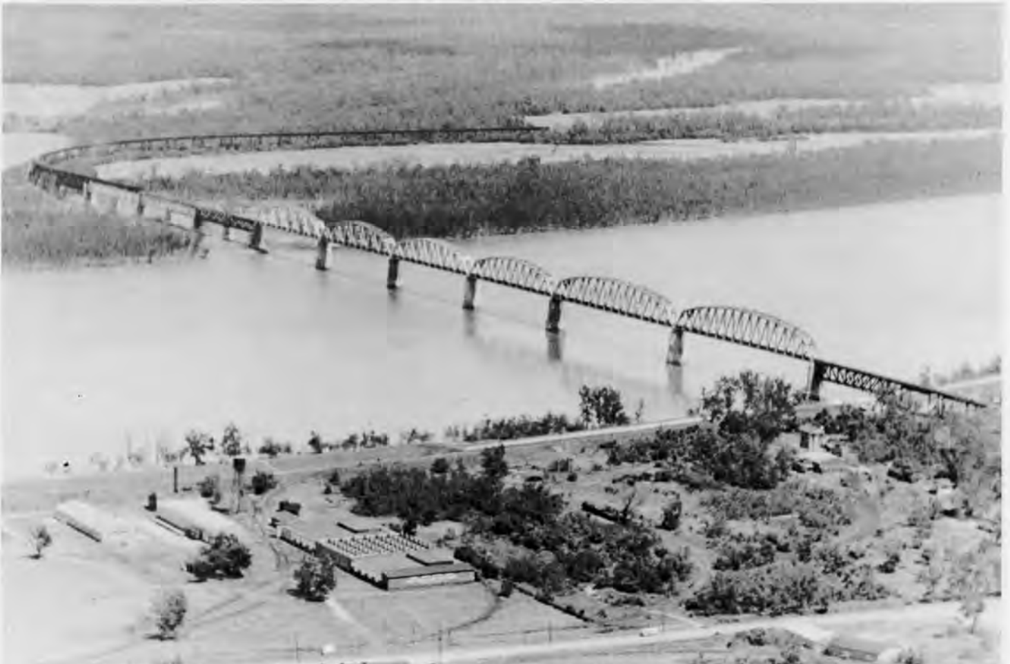
This aerial view from the Illinois side of the Ohio looking across the river to Kentucky shows the new bridge and the long trestle approach on the Kentucky side. ICRR photo.
