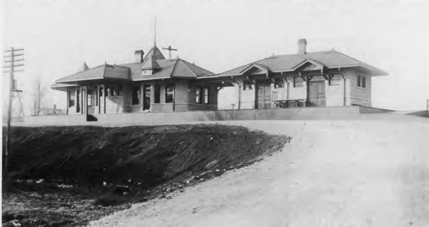
In this northeast view, the baggage express room can clearly be seen. This is the only portion to survive, and is now a Japanese restaurant. ICRR photo Author's collection.
