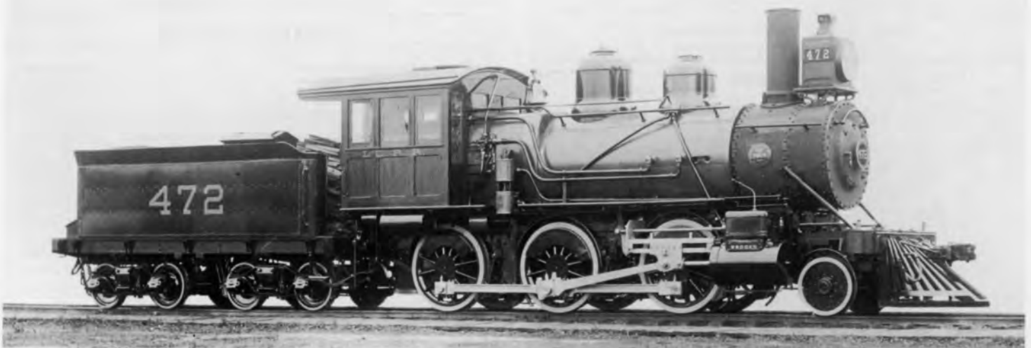
#472. A Brooks portrait in November of 1895 serves as a reminder of how these Mogul types looked at the turn of the century. The Belpaire-fired #472 was assigned to the Indiana Division until sold in 1929, so far as known. Alco Historic Photo Author's Collection.
