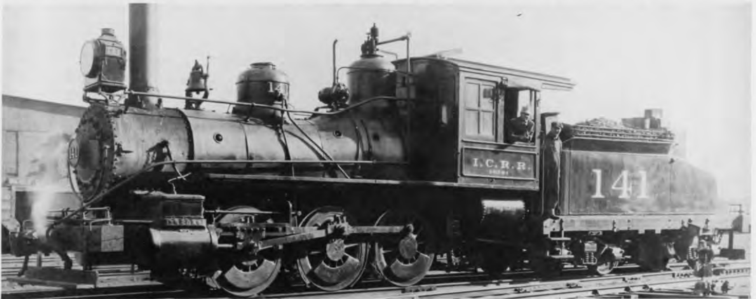
0-6-0 #141, built by Brooks in 1893. 18"x 24" cyl. 51" dr. scrapped in 1925. ICHS photo
